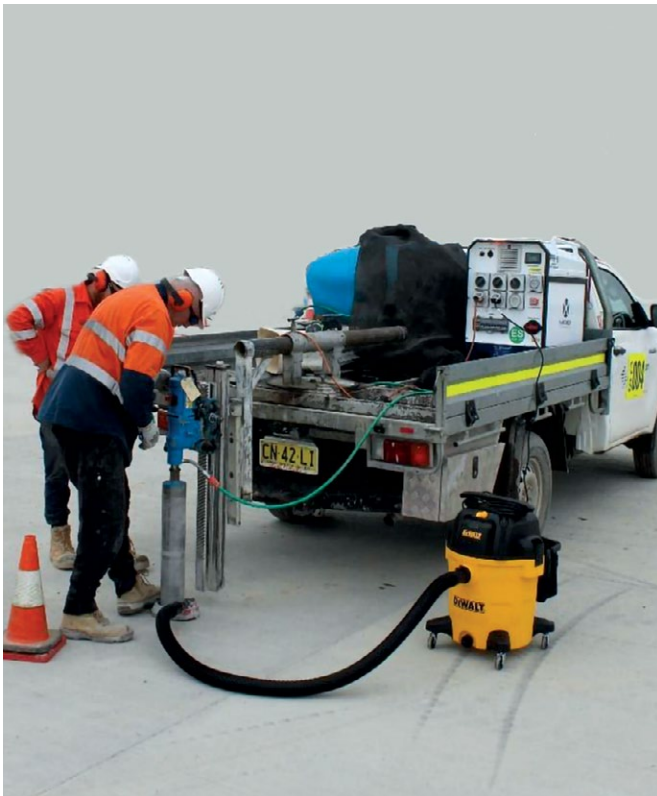
PPB 8-15 Concrete Coring
