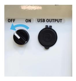
2. Further to the above, switch off all the circuit breakers (push down) and isolator. The isolator is shown below in the "ON" position. Rotate anticlockwise 90 degrees to turn to "OFF" position.
